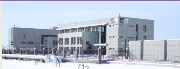
Tianjin plant (est. since Sept., 2005)
