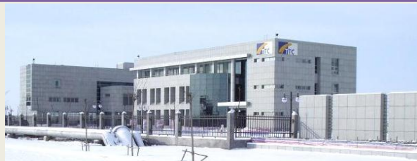
Tianjin plant (est. since Sept., 2005)
